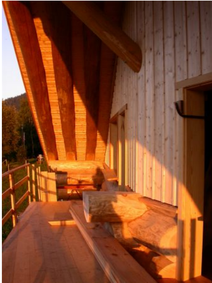
Balcony (1st floor) Valley side
