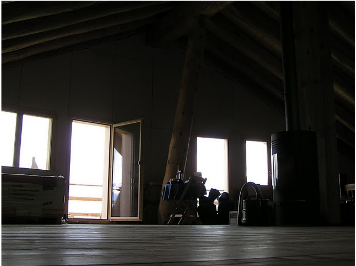
Loft space upstairs
