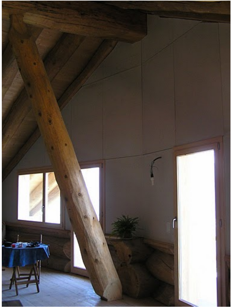
Valley side upstairs
